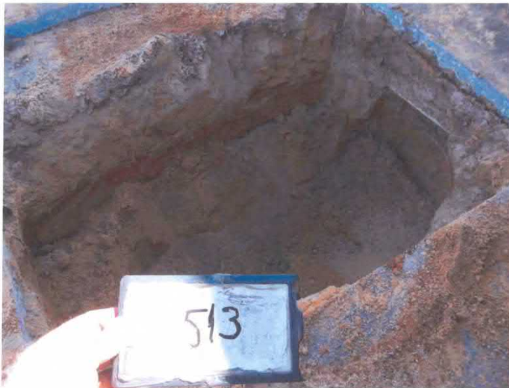
Picture 2: UST 513LaurelBB excavation.
