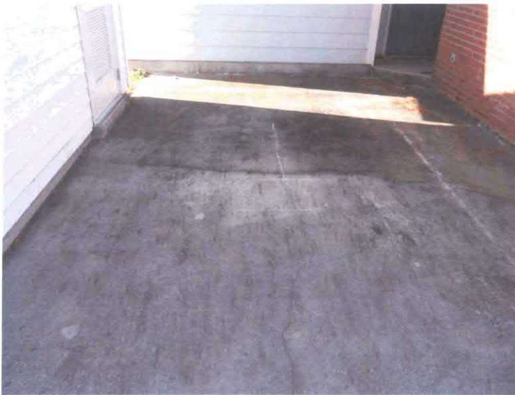
Picture 1: Location of UST 513LaurelBB.
